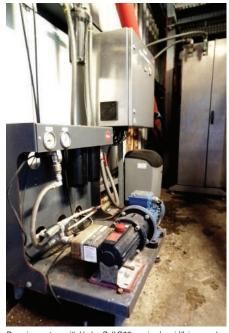
Pumping system with Hydra-Cell G03 serving humidifying nozzles. This pump replaced a 'high-maintenance' piston pump at the plant.
